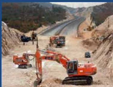
Construction of the Bar - Boljare highway
